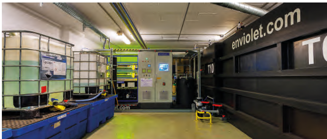
Figure 8: UV oxidation plant at a softgel factory: On the right the storage and batch treatment tanks can be seen and the UV reactors and the electrical cabinet with the fully automated process control are at the rear. Chemical storage is on the left. The SOP makes the system adaptable to a changing wastewater matrix. The modular design also allows for relatively easy upscaling to handle, e.g., larger wastewater volumes.
